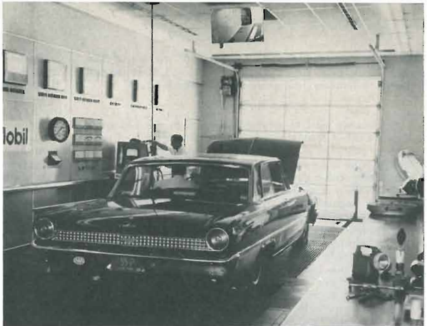
Fig. 1. Typical drive-through diagnostic lane. The cars enter one end where the dynamometer is located (note view in mirror hanging from ceiling), and after these tests, car is further tested at this second location. Note large readout meters on the wall.
