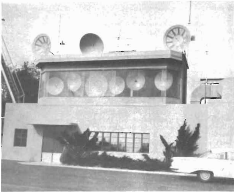
Fig. 3. Weather-shielded microwave antenna housing for studio-to-transmitter microwave relay, photographed at Mt. Wilson, Calif.
